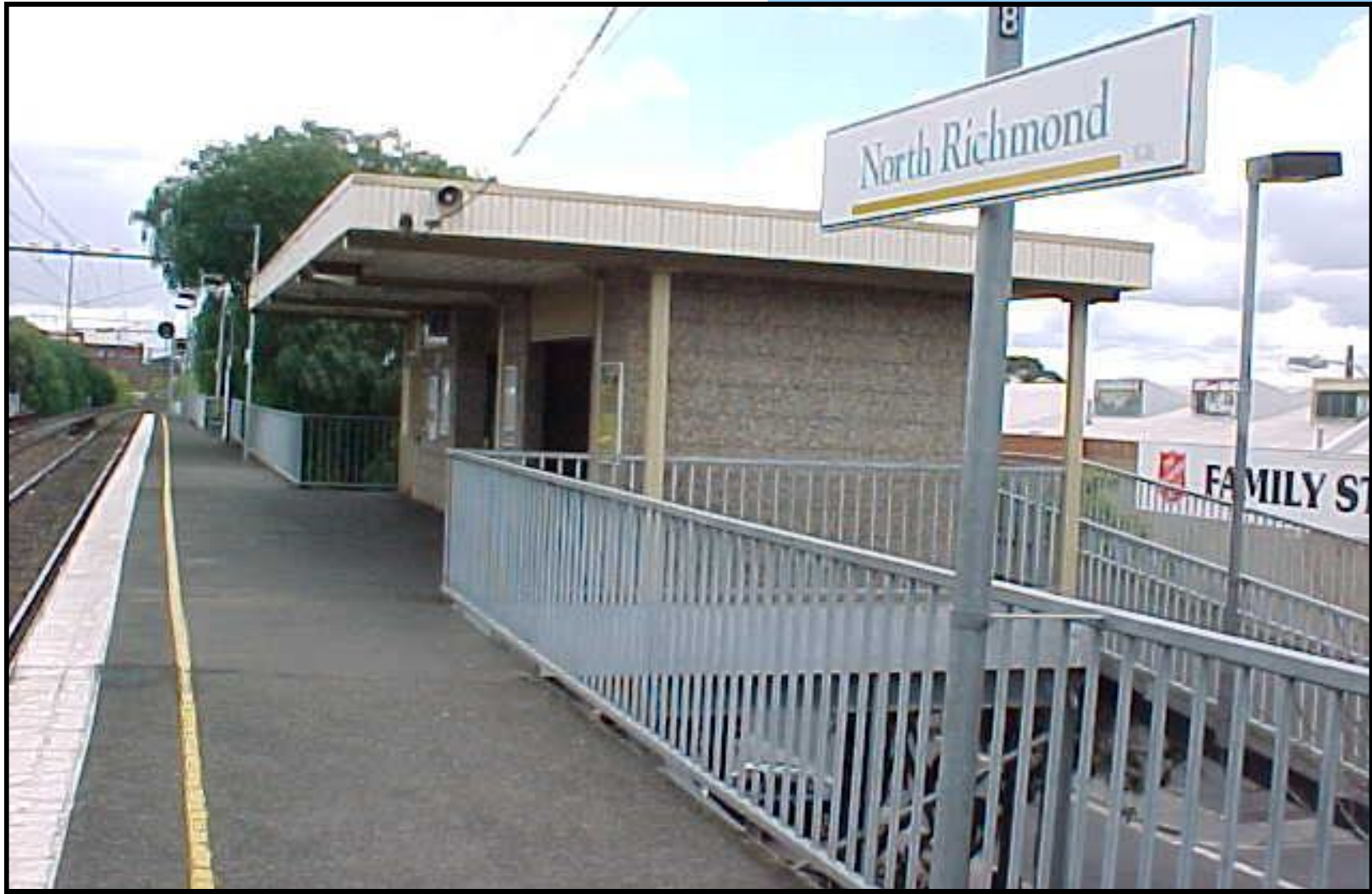
Figure 5.N Zare.North Richmond Station.2024
