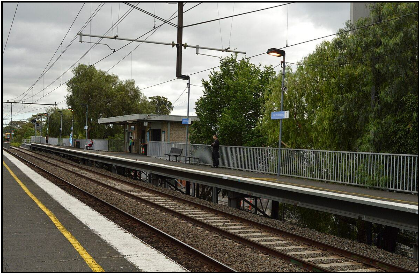
Figure 4.N Zare.North Richmond Station.2024
