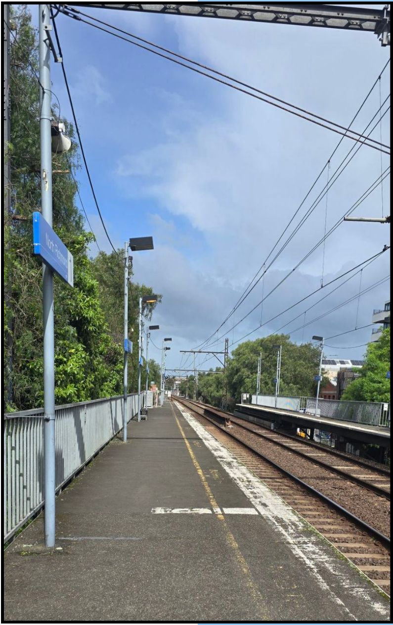
Figure 3.N Zare.North Richmond Station.2024
