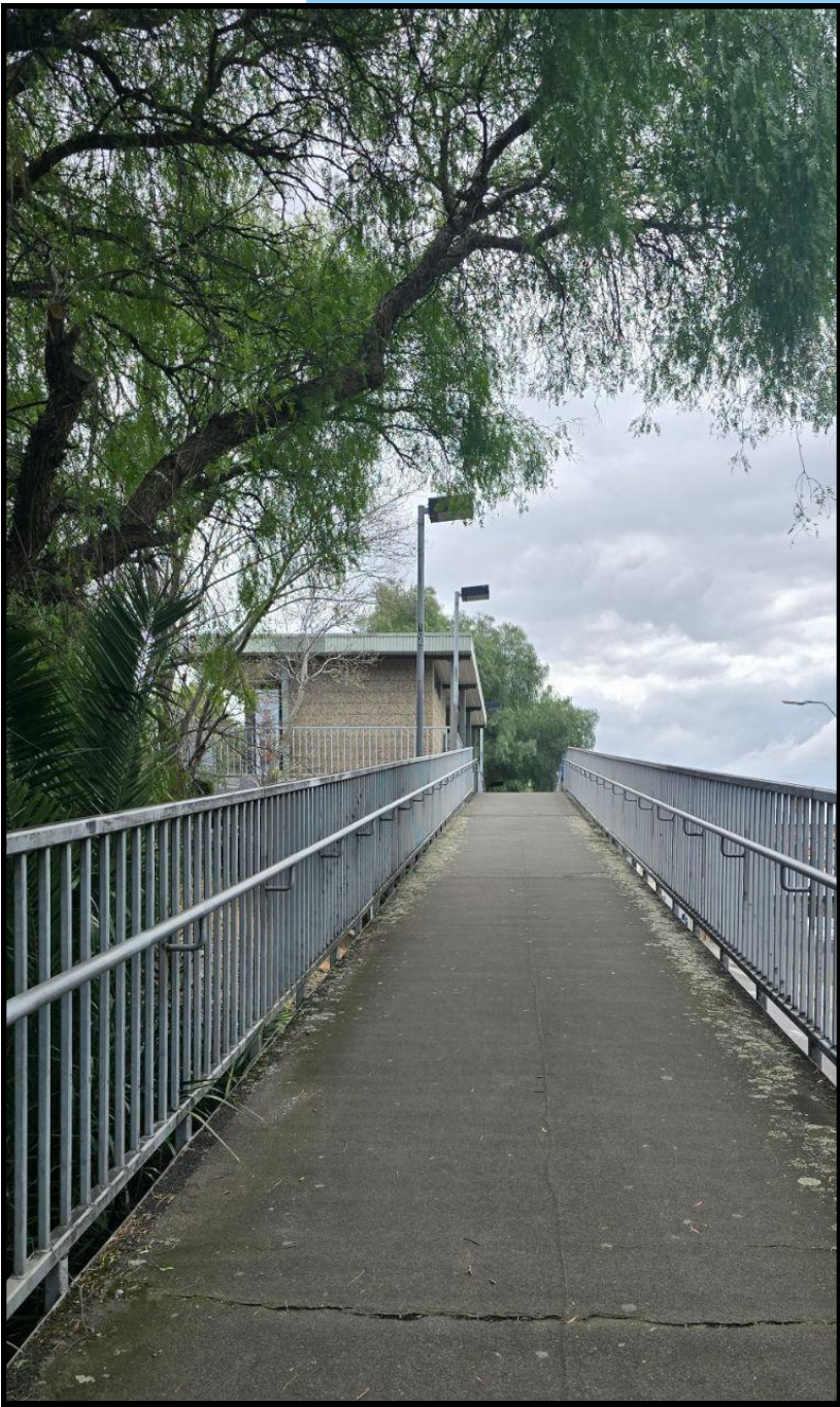
Figure 7.N Zare.North Richmond Station.2024
